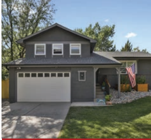
Villa Loma COLORADO SPRINGS, CO 80917
